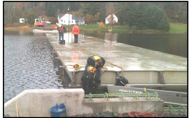
**Figure 10: Onsite construction; diver onsite for field connections.**
