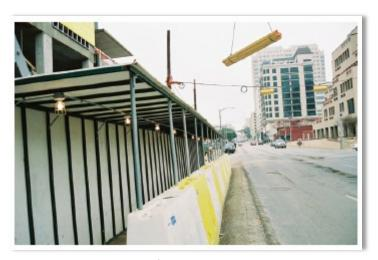
A covered walkway protects pedestrians from construction dangers occurring above them including falling debris. Covered walkways shall be lit for nighttime use and include proper barriers along their alignment.
