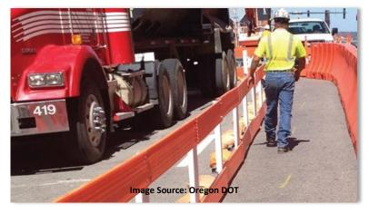
Above, the pedestrian route is delineated on both sides to provide a physical barrier between the pedestrian and the work zone as well as between the pedestrian and vehicle traffic.
