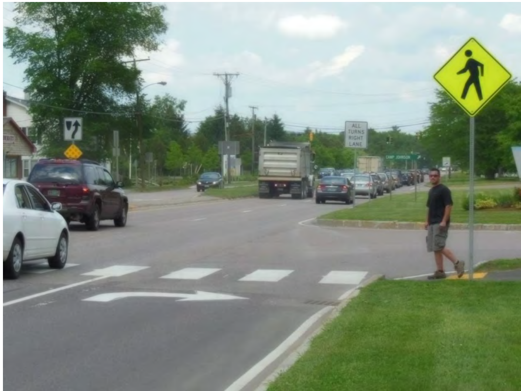
Figure 3. Looking and stepping crossing scenario, pre HAWK installation.
