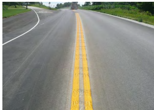
Figure 10: Centerline rumble stripes immediately after painting in Sheldon, VT.
