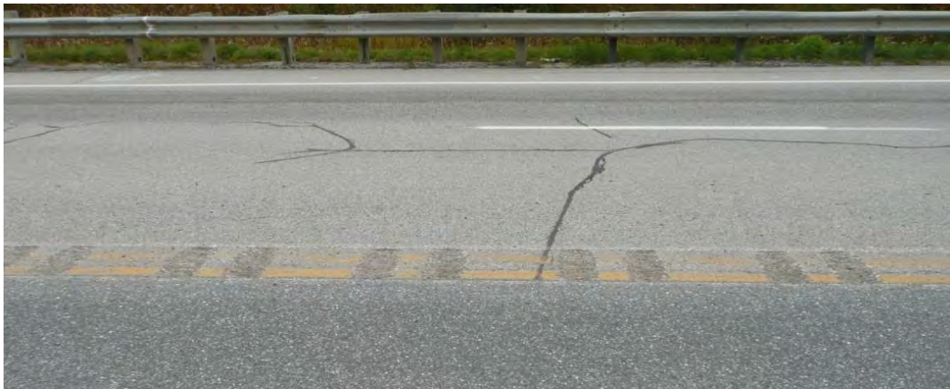
Figure 8: Rumble stripes after milling and sweeping.
