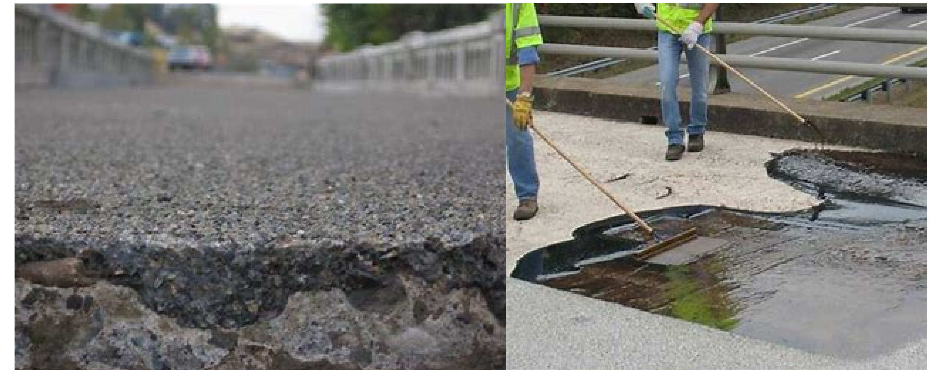
Figure 3. Polymer Deck Overlay
