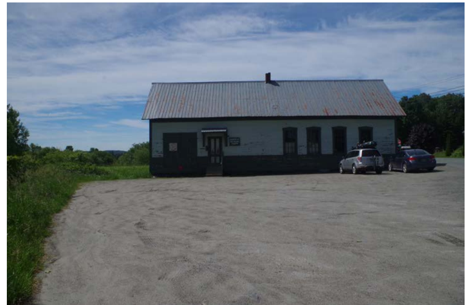
Parking at the old train station on Peacham Road
