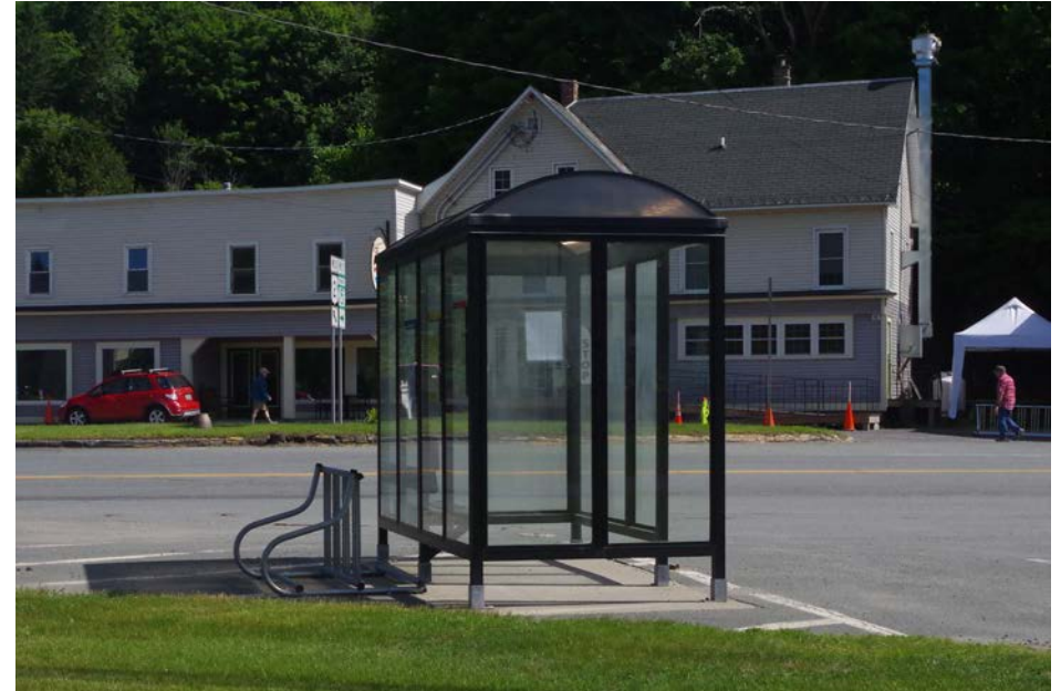
Bus stop in the West Danville Park & Ride with bike parking
