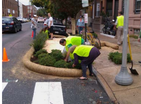
Philadelphia, PA - Temporary curb extensions Image from Project for Public Spaces
