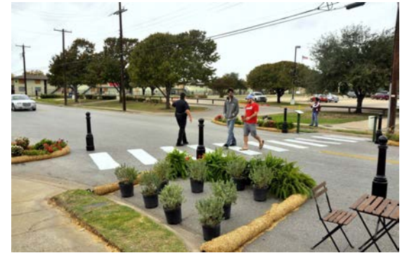
Dallas, TX - Temporary curb extensions Image from Project for Public Spaces
