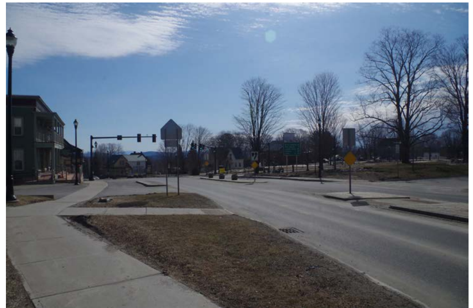
Sidewalks and crossing of Route 2 with a raised median in the Village
