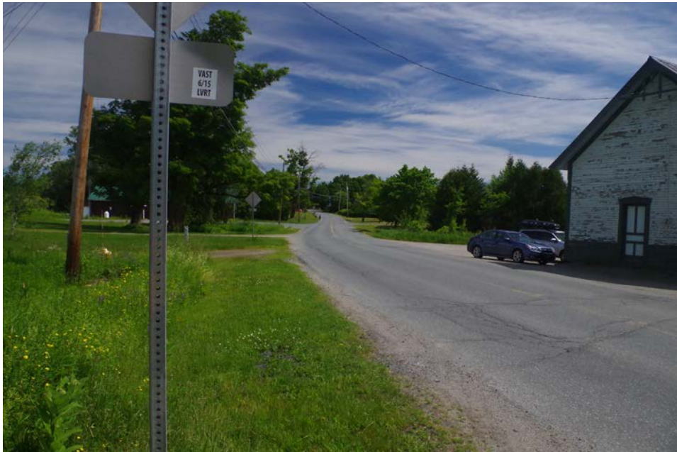
Looking north at the train station on Peacham Road
