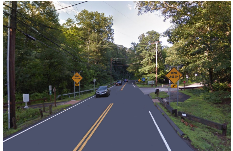
Rendering of a rail trail crossing with upsized signs that are gate-posted Canton, CT. Original image from Google maps
