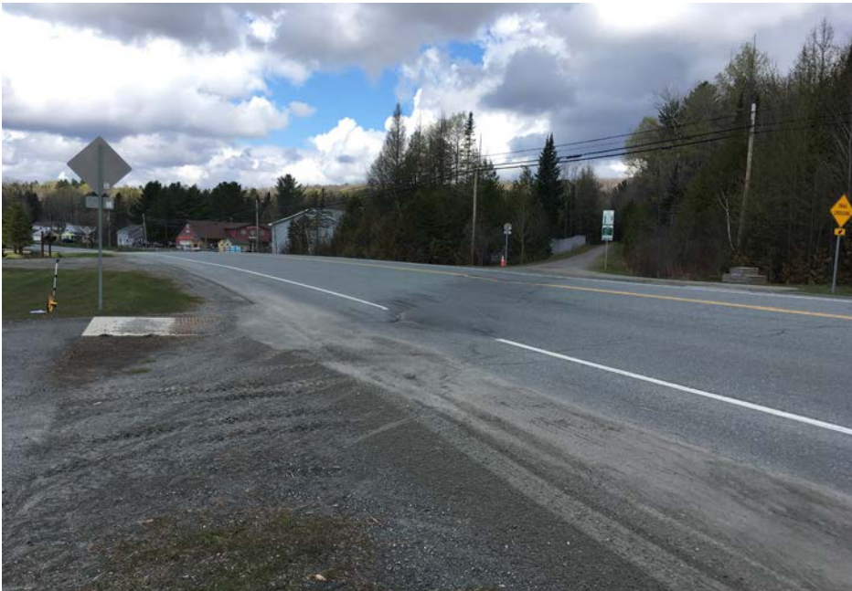
Route 2 crossing near Larrabee's (looking west)
