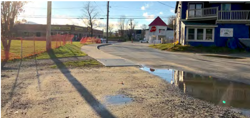
Impervious surface and a poor drainage pattern creates pooling on Mill Street.
