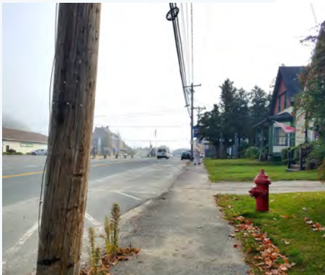
Asphalt sidewalks are level with the roadway. With no striping they look just like the road or shoulder.
