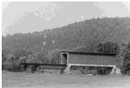
Cambridge Junction, Br 68 113' span Built 1899, replaced 1967
