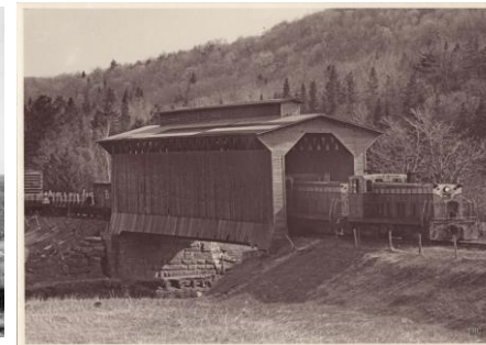
Fisher Bridge, Wolcott 103' span Built 1908
