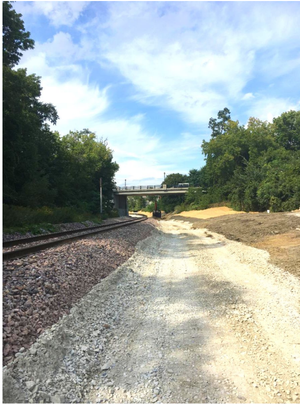
Kubricky crews are constructing a utility access road on the south end of the project.
