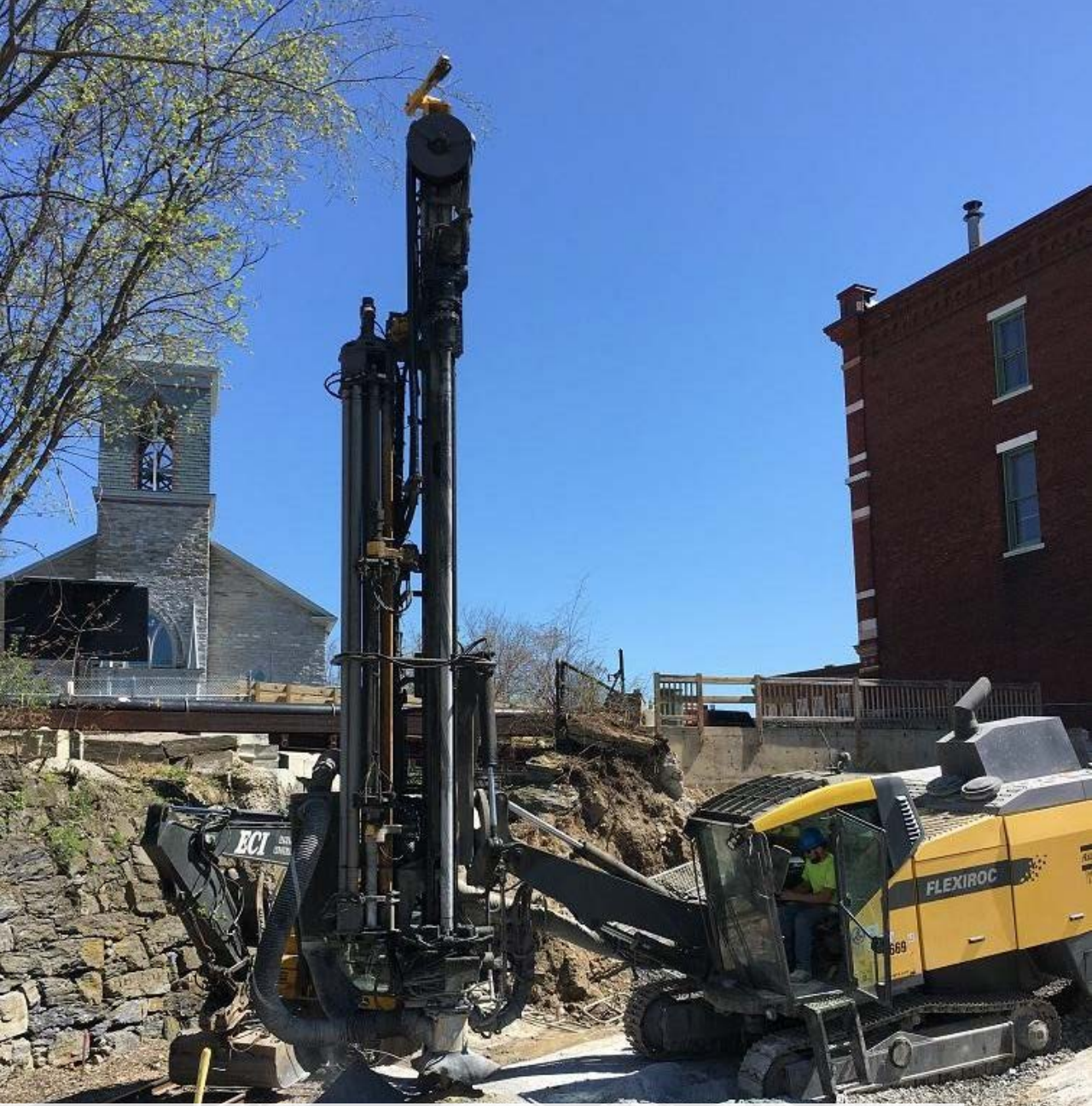
Microtunneling Launch Shaft Construction
