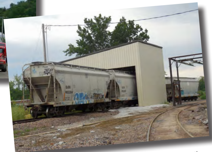
The track for this transload facility in the Burlington rail yard was built with a three-way cost-sharing, one third by the customer, one third by Vermont Railway and one third by the State.
