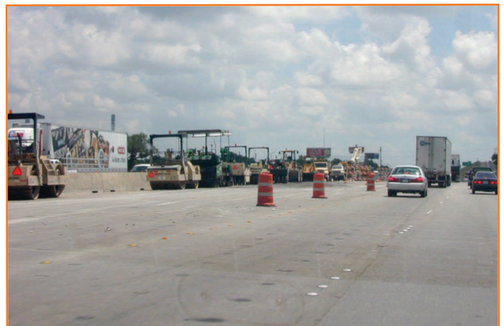
Some work zones include a large distance separating the traffic space and work space (Source: TTI).
