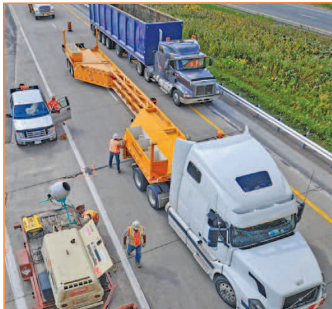
Highly-mobile barrier systems deflect very little when hit by an errant vehicle (Source: QMB Barrier).
