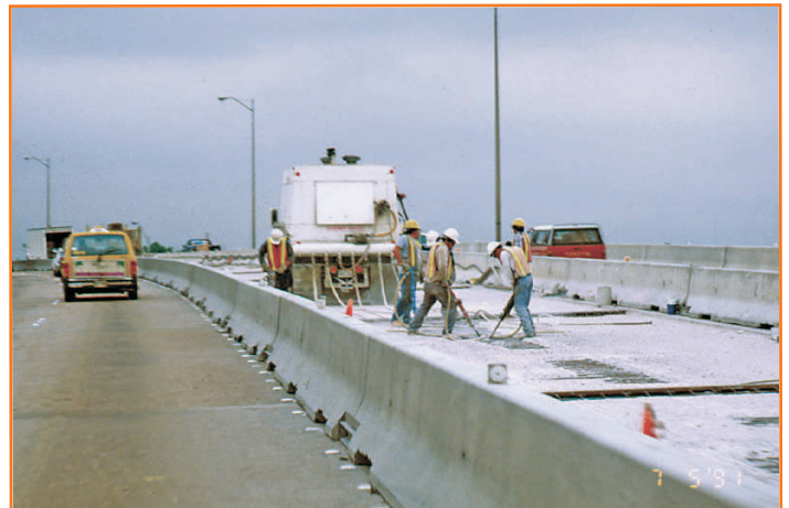
Some work zones include concrete barriers to separate the traffic space and the work space (Source: TTI).
