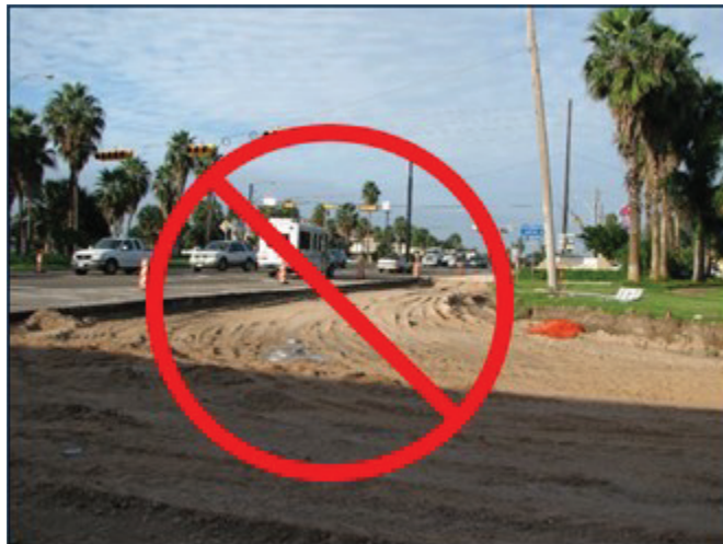
Figure 4. Sidewalks should not lead directly into unprotected work spaces (source: TTI)
