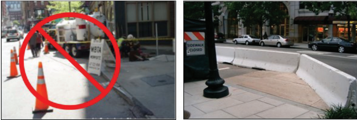
Figure 15. Proper separation devices must be used when diverting pedestrians into travel, parking, or bicycle lanes (Source: J. Barlow, Accessible Design for the Blind; TTI )
