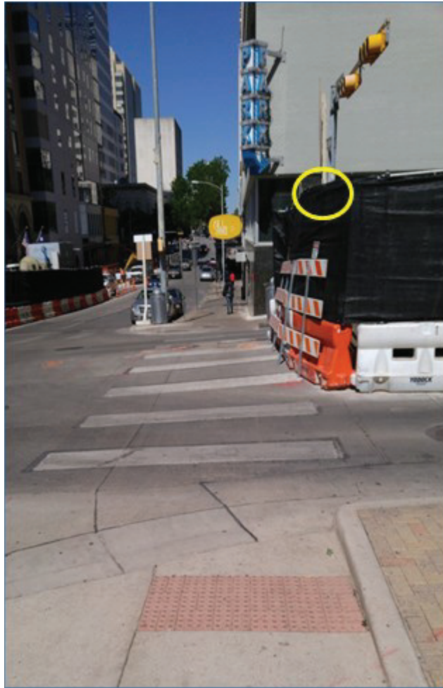
Figure 6. Work zone devices and materials can obscure pedestrian signals can make it difficult for pedestrians and right-turning vehicles to see each other (Source: FHWA)
