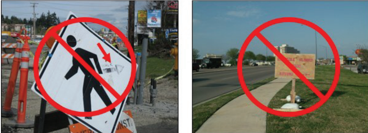
Figure 17. Hand drawn signs or modifications to signs are not appropriate for detouring pedestrians (Source: TTI)
