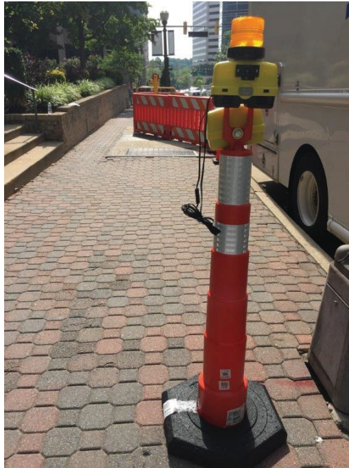
Figure 10. Audible pedestrian warning devices should be carefully positioned and use good message design principles (source: Virginia Department of Transportation)
