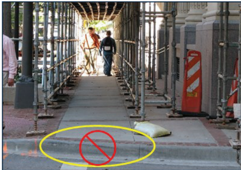
Figure 13. Proper temporary curb ramps are required wherever the diversion path traverses a curb (Source: TTI)
