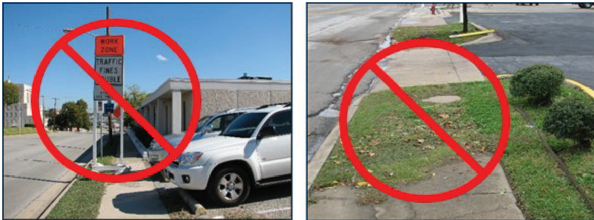
Figure 19. The pedestrian detour route should be continuous and free of obstacles (Source: TTI)
