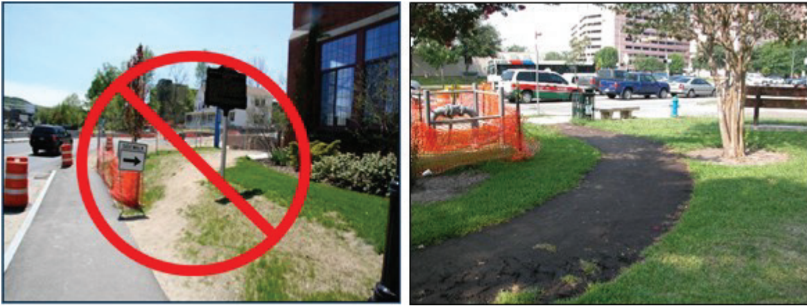
Figure 12. Diversion paths should be smooth, solid, weather resistant, and detectable by visually-impaired pedestrians (Source: TTI)
