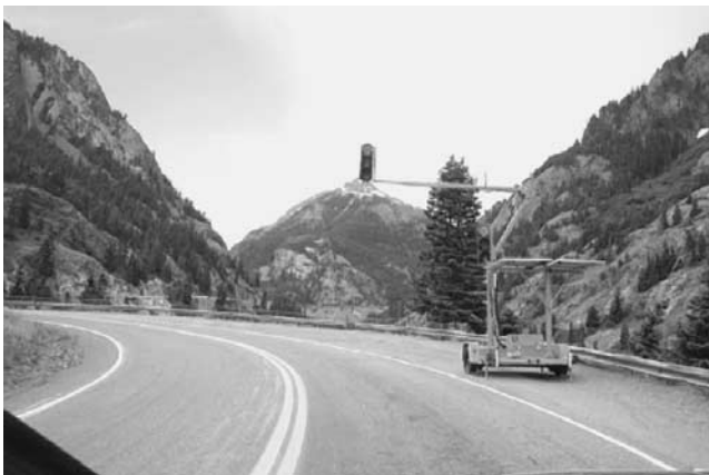
Figure 20. Temporary traffic signals.
