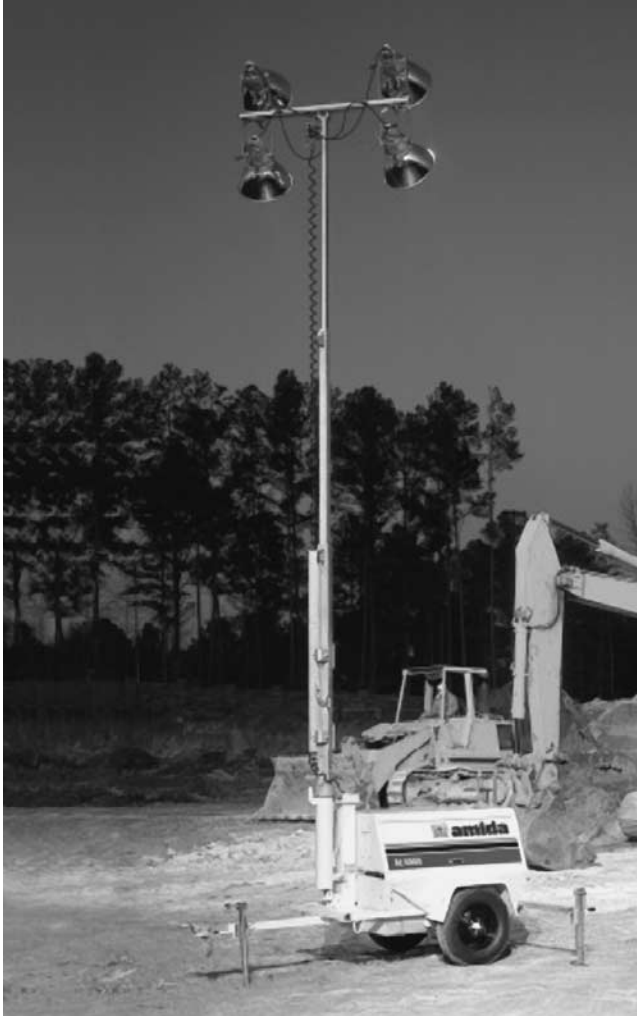
Figure 32. Portable trailer-mounted light tower raised into position at the work site.
