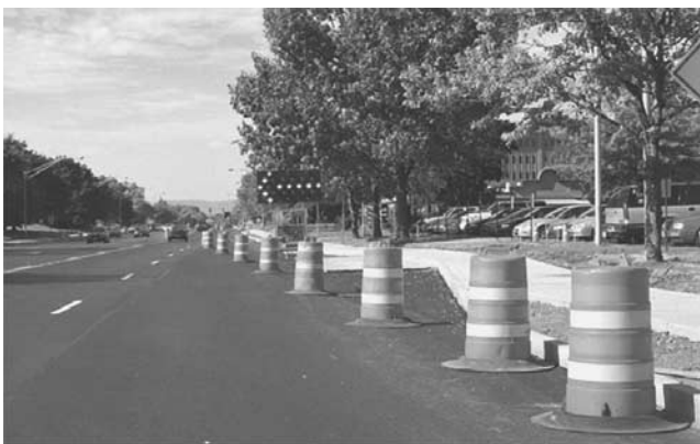
Figure 1. Lane closure taper.
