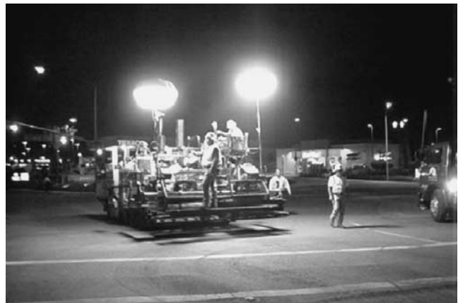
Figure 29. Light balloons attached to pavers and other equipment.
