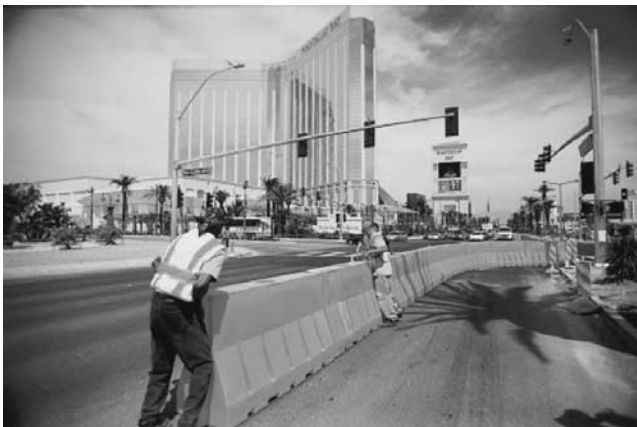
Figure 18. Portable plastic barrier, which requires no heavy equipment for placement.
