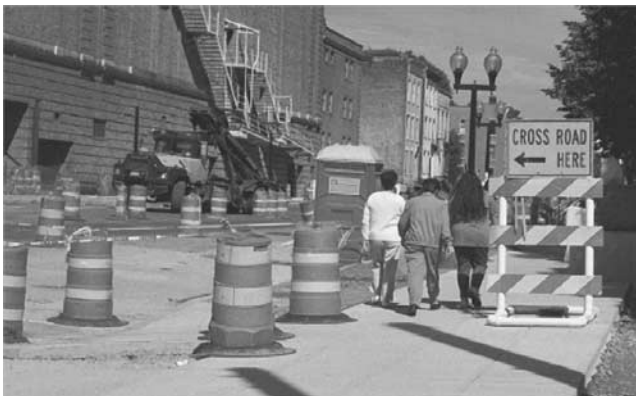
Figure 4. Clearly marked, temporary pedestrian paths.
