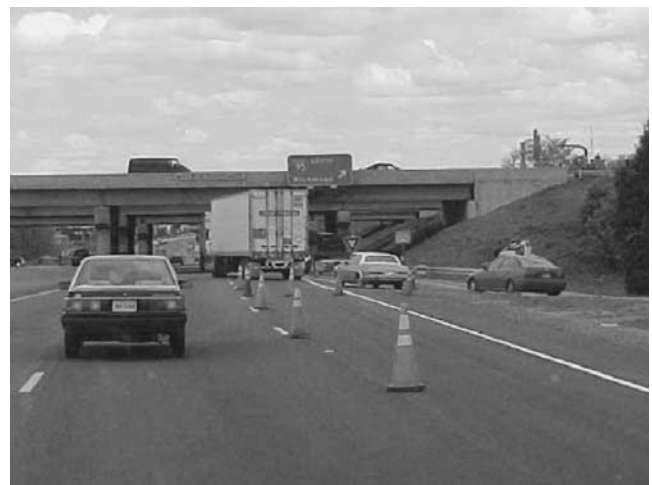
Figure 10. Closely spaced cones during the day.
