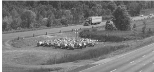
Figure 38. Equipment safely stored in median beyond the roadside clear zone.
