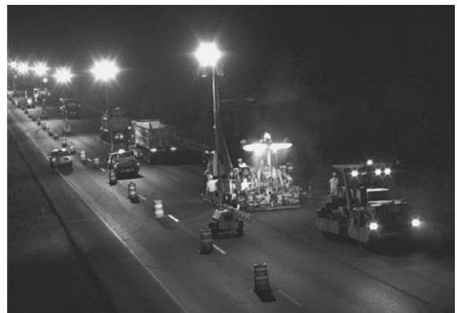
Figure 28. Level I and II illuminance at a nighttime paving project.
