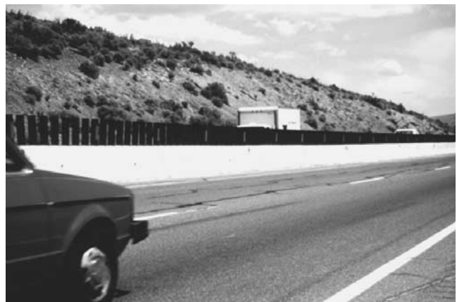
Figure 22. Screens mounted on temporary traffic barrier.
