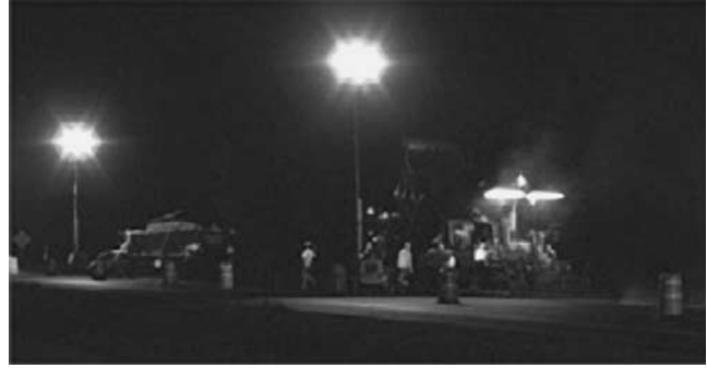
Figure 33. Supplemental flood lights mounted on equipment.
