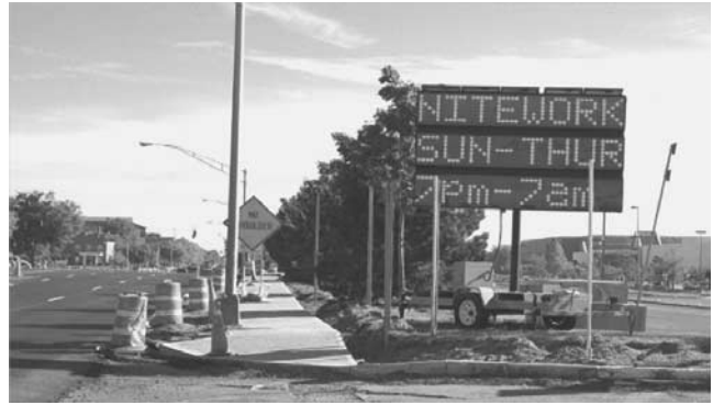
Figure 15. Changeable message signs communicating night work schedule.
