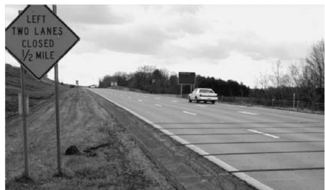
Figure 21. Temporary rumble strips formed from removable pavement masking tape.
