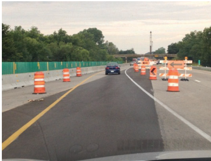
Figure 5. Use of Paint on Lane Shift on I-44 in Oklahoma.
