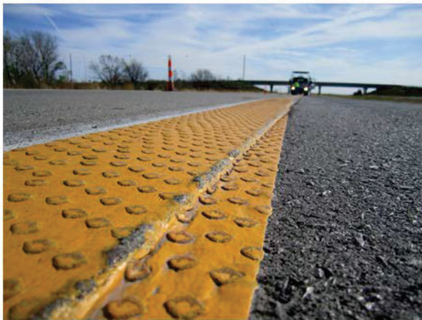
Figure 6. Pavement Marking Damage in a Work Zone
