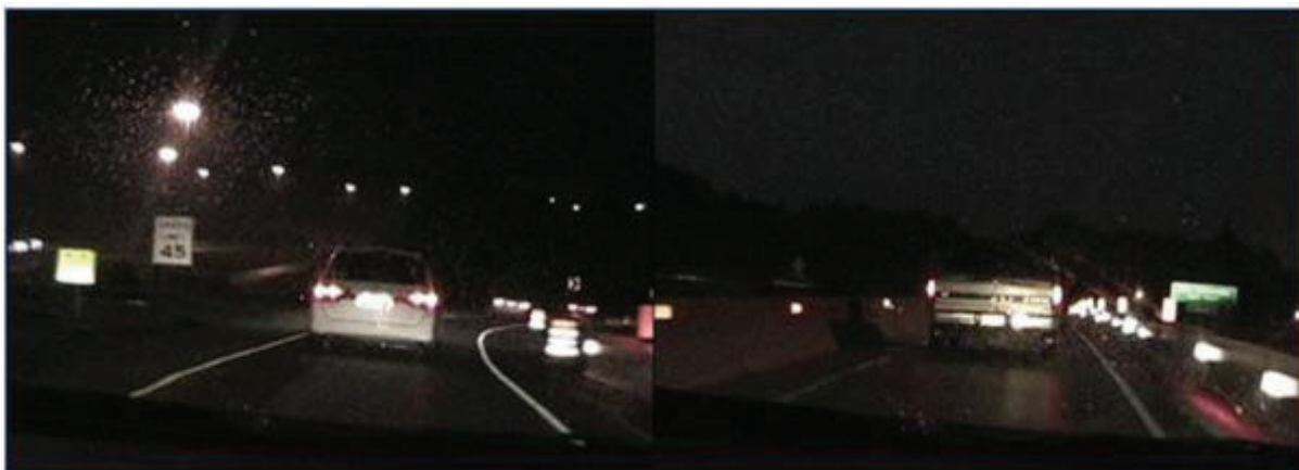
Figure 8. All-weather Pavement Marking (left) and Standard Pavement Marking (right) Work Zones on US-32/33/50 Eastbound in Ohio (Nighttime).
