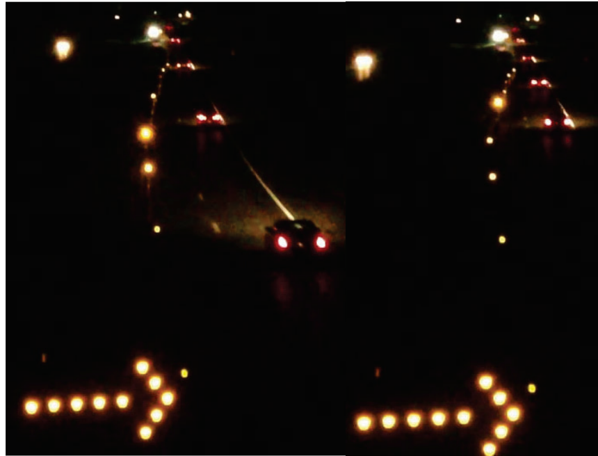
Figure 16. Sequential Work Zone Taper Warning on US Route 54 in Missouri.
