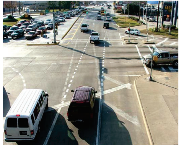
Figure 13. Removed Markings ("Ghost Markings") Compared to Existing Pavement Markings (Source: Texas Transportation Institute, 2008)
