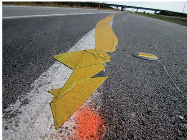
Figure 6. Pavement Marking Damage in a Work Zone
