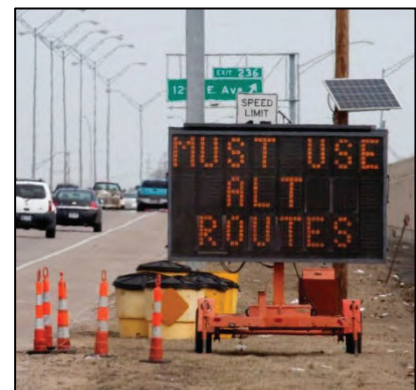
Figure 19 – PCMS Warning Drivers to Find Alternate Routes around the Work Zone 11
