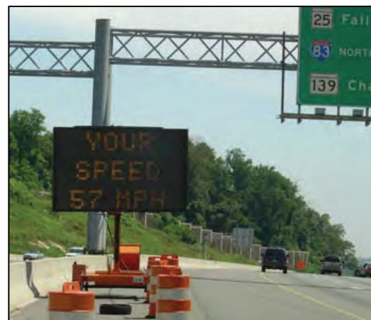
Figure 15 – PCMS Displaying Speed of Passing Vehicles in a Work Zone 8
