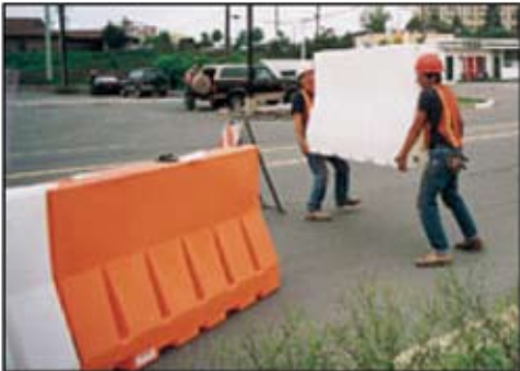
Figure 3. Empty Ballast-Filled Barrier Segments
