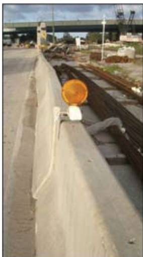
Figure 1. Portable Concrete Barrier Separating the Traffic Space and Work Space
