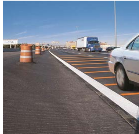
Figure 9. Orange adhesive rumble strips. (Source: Advanced Traffic Markings, 2013)
