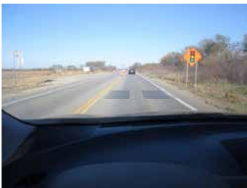
Figure 10. Wheel path rumble strips (left) and continuous rumble strips (right).
