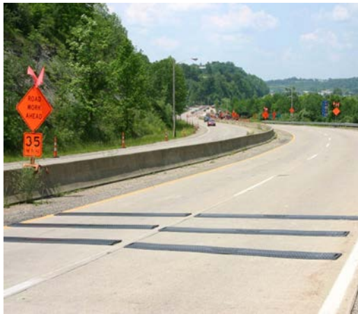
Figure 1. Temporary rumble strips applied on the approach to a work zone.
