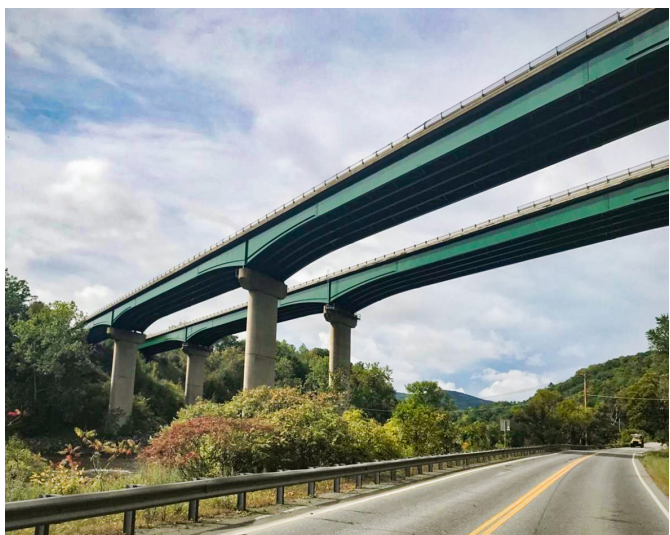
SHARON. Bridge repairs along I-89 over the White River in Sharon were completed this year. Work included rehabilitating both bridge decks with all structural steel stripped and recoated.
