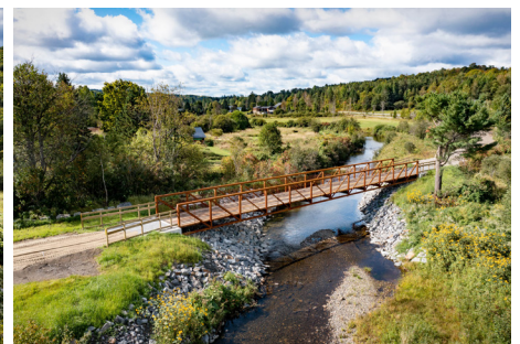
New trail bridge in Greensboro Bend.
