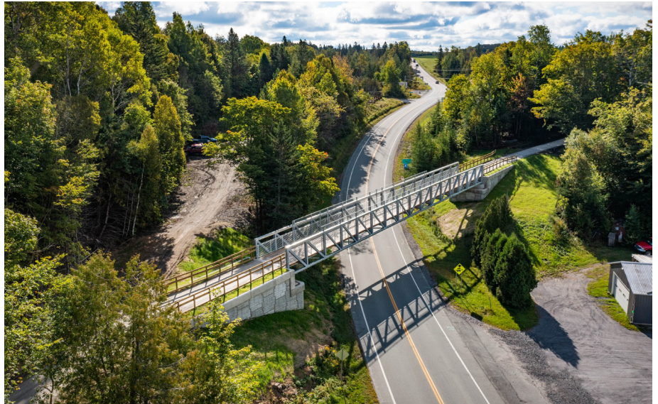
A new rail trail bridge was installed over VT Route 15 to connect segments of the LVRT in Walden.
