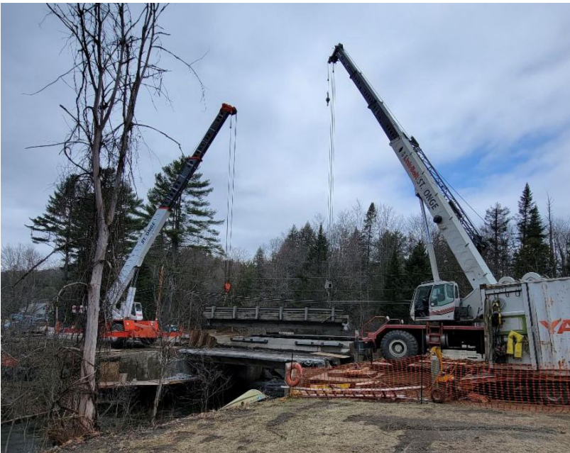
CALAIS. A series of bridge replacements continued on VT Route 14. With Bridge 74 completed in 2021, work began on Bridge 77 and Bridge 82, both over the Kingsbury Branch of the Winooski River. Originally built in the 1910s-1920s, all three bridges required significant work to be brought up to modern standards. Bridges 74 and 82 were completely replaced, while Bridge 77 underwent a deck and superstructure replacement but kept the existing substructures due to its better condition. The new expected service life of Bridges 74 and 82 is now 75 years, with the the superstructure of Bridge 77 projected at 40 years.
