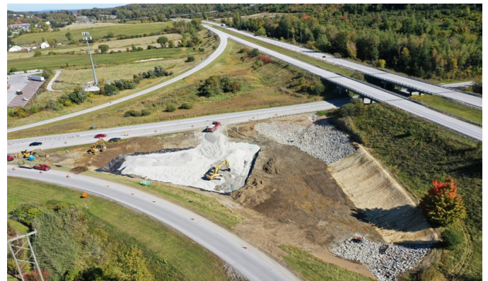
FIGURE 3. Drone imagery of Exit 19 on Interstate 89 in St. Albans.
