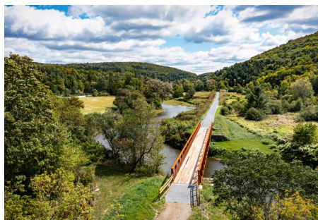
Completed LVRT bridge in Wolcott.
