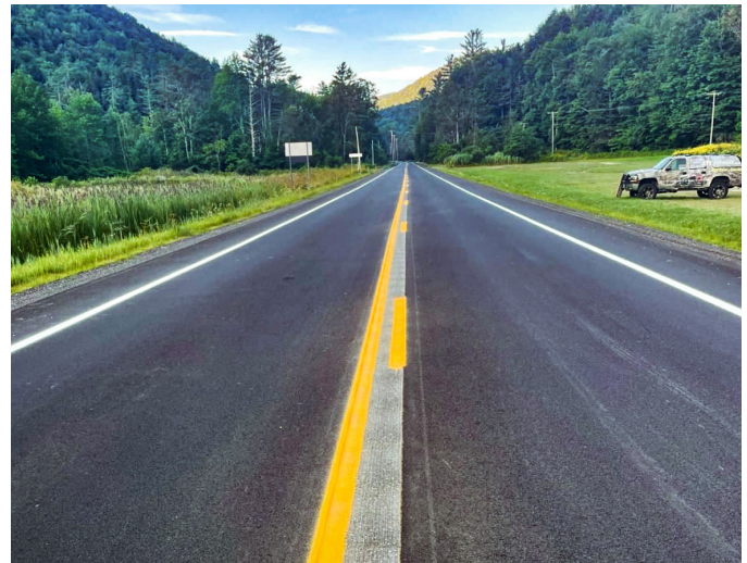
PLYMOUTH - BRIDGEWATER. It was a busy summer along VT Route 100 as crews completed 16 miles of paving, replaced guardrail, and installed rumble strips on the roadway.
