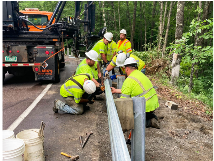
FAYSTON. Many maintenance projects require collaboration among different district garages, like this guardrail repair along VT Route 17 that saw three different crews team up to remove, replace, and clean up the project area in one efficient afternoon.
