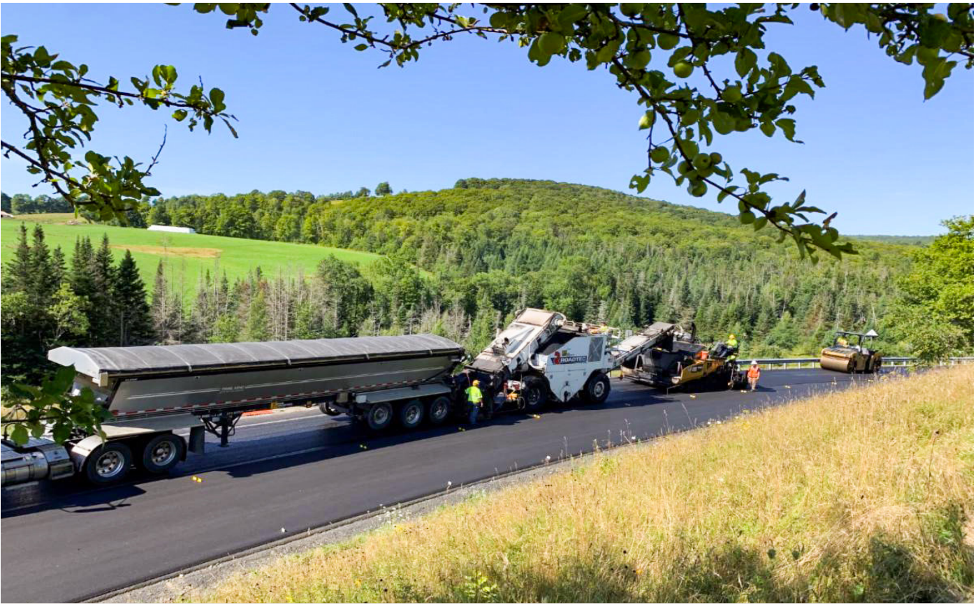
CHELSEA - THETFORD. In 2022, a 15-mile paving project on VT Route 113 was completed. The project included a full-depth reclamation of the roadway, superelevation correction, new guardrail, improved signage, drainage, and more.
